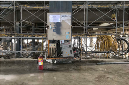
Preventing electric shock by elevating the electrical wires and electric boxes.
