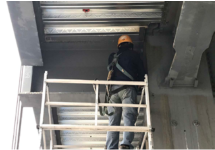
Ensuring that staff wear safety harness when working at height with lanyard anchored to the guard rail.
